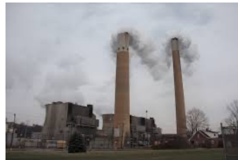
Coal fired power plant
